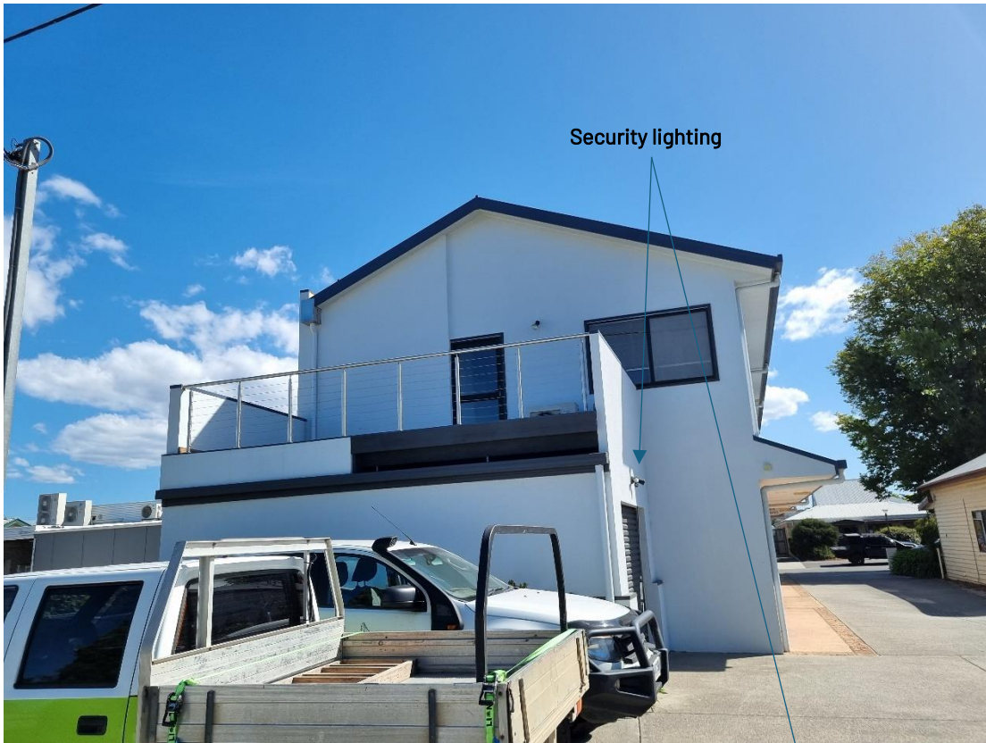
Figure 5 Rear of building and garage/ car parking
