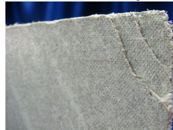
Asbestos cement panel
