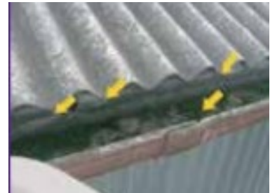
Cement roofing and gutters
