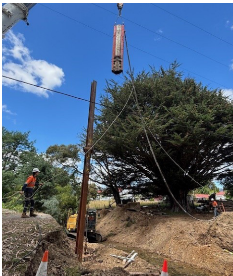
Photo: Working on the bridge replacement at Mangana.
