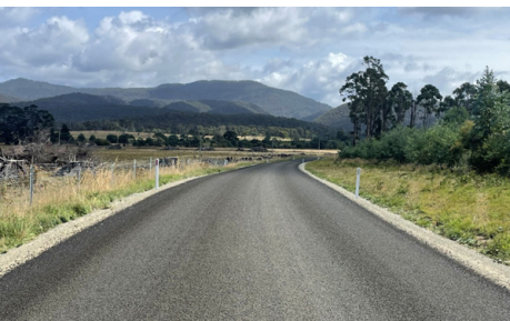
Photo: Mangana reconstruction works
