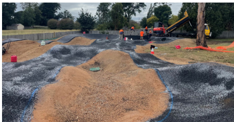
Photo: Fingal Pumptrack under construction
