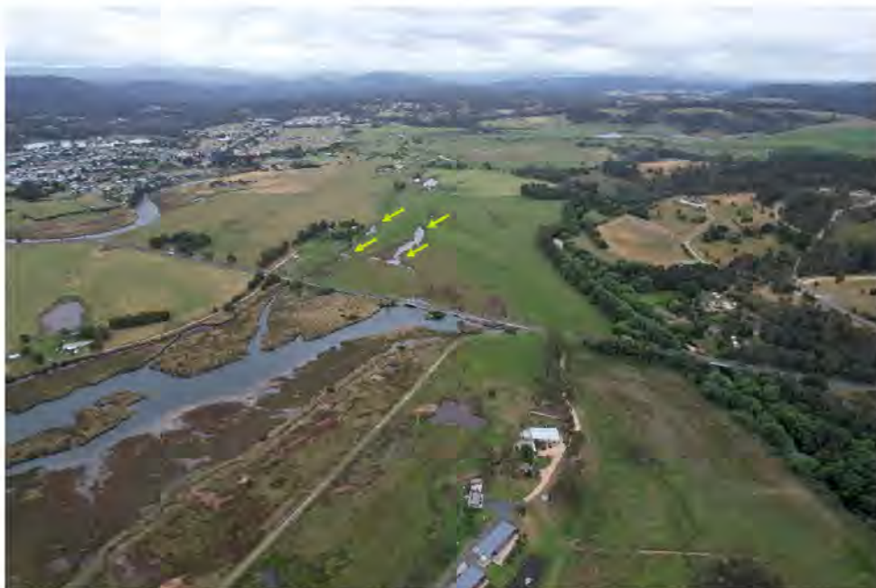
Figure 4. Aerial view of the salt marsh at the edge of Georges Bay which is separated from the George River floodplain by Binalong Bay Road. Yellow arrows indicate scour channel shown in Figure 5.
