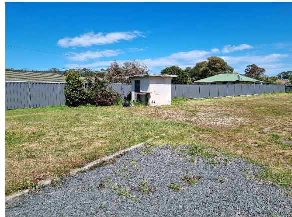
Figure 3 rear of dwelling looking south west
