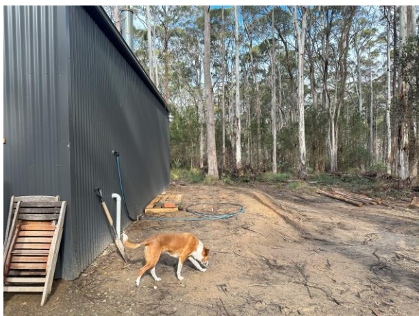
Potential location for the firefighting static water supply – western side of existing shed
