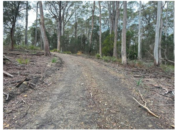
The top part of this section is greater than 10° and will need to be sealed for this small section
