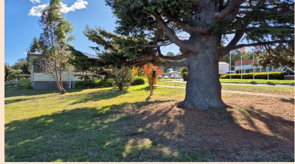
Existing fire plug
