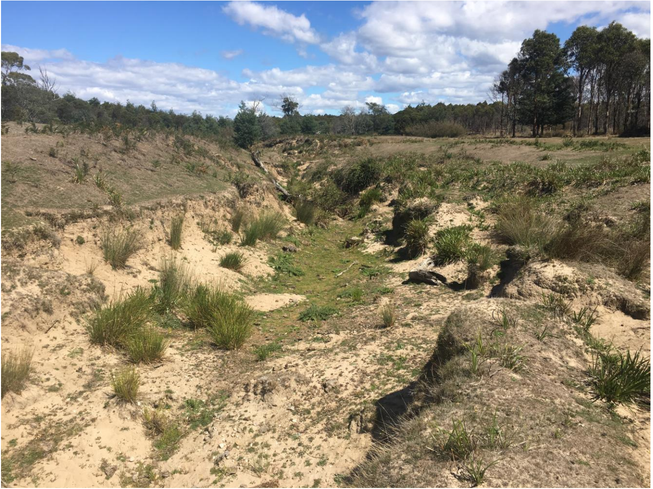
FIGURE 2-9 THE AVULSION FLOW PATH NEAR PRIORY.
